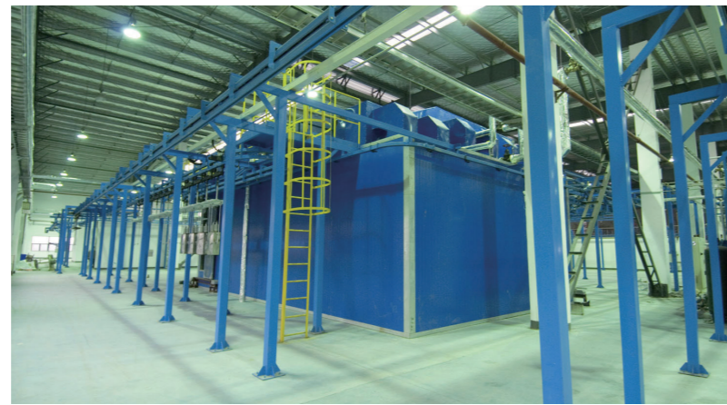
Hot drying leak testing furnace
