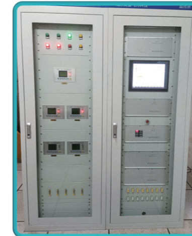
Diagram of the 125 MVar/33 kV SVC Unit of Tianjin Steel Pipe Co., Ltd.
